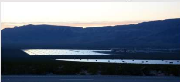
Figure 5.2-1. Black PV Panels at CM 1 and 2 Facilities Appear White When Low-Angle Sunlight is Reflected from the Panels (Background), and the PCU's look black.
